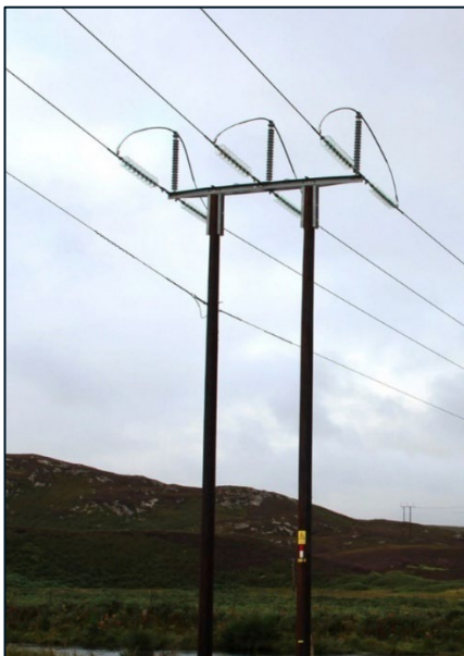
Figure 1-3 Indicative wood pole design for Overground Inter-Array
